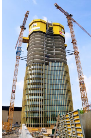
Figure 7 and 8: Transfer of the chosen geometry in a project coordinate system and by a geometer on the construction site.
